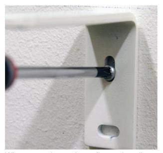
When mounting to the wall, attach wall mounting brackets to the wall.
