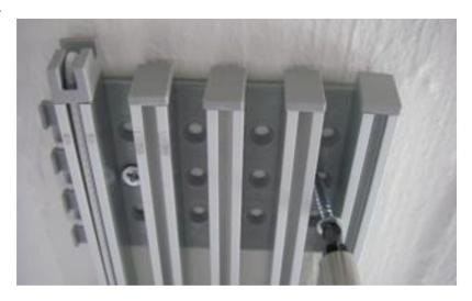
When mounting to the ceiling, attach the fix plates directly to the ceiling. The fixplates must always be attached from both ends.
