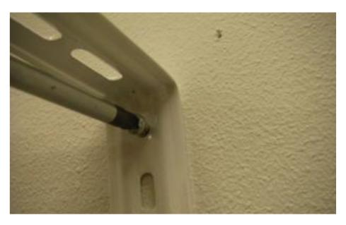
When mounting to the wall, attach wall fixing brackets to the wall.
